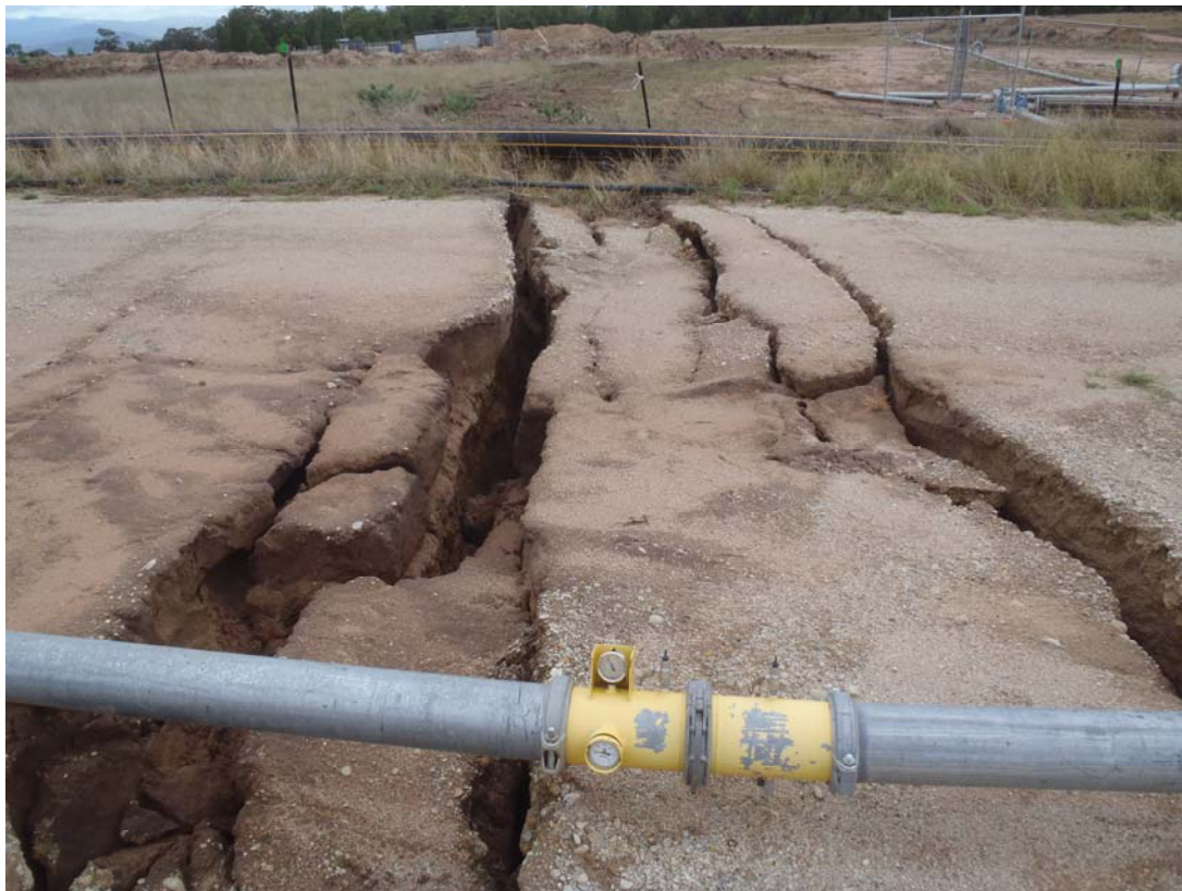
Photo 2: Surface Crack in LW104
